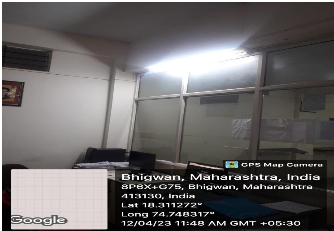
Geo-tagged photograph of use of LED tubes in administrative office on ground floor.
