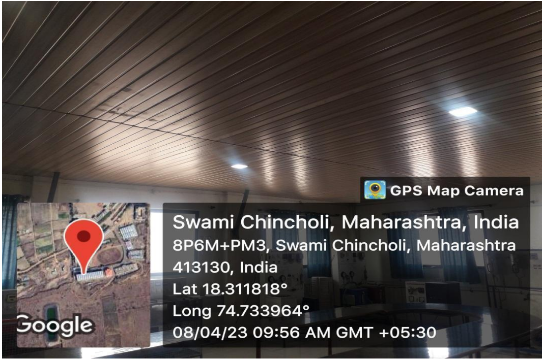
Geo-tagged photograph of use of LED Bulbs in RAC Lab of Mechanical Department.
